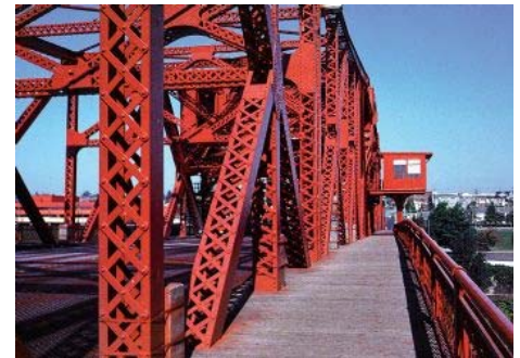
Image courtesy of Jim Martin Public Works Photo Library at www.apwa.net .
