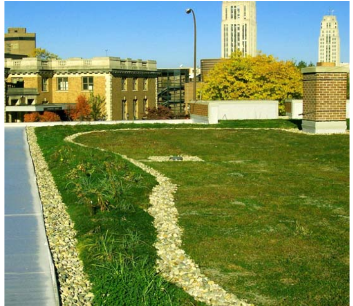
The City of Battle Creek, Mich., Public Safety Building's green roof was named a 2006 Public Works Project of the Year by APWA. Awarded in the Structures category, less than $2 million range, the 18,000-square-foot vegetated green roof atop the City's Public Safety Building is believed to be the first of its kind in southwest Michigan. A lightweight, layered system covering waterproofed roof surfaces, the building's green roof has growing vegetation including drought-tolerant succulents, grasses and native flowers.
