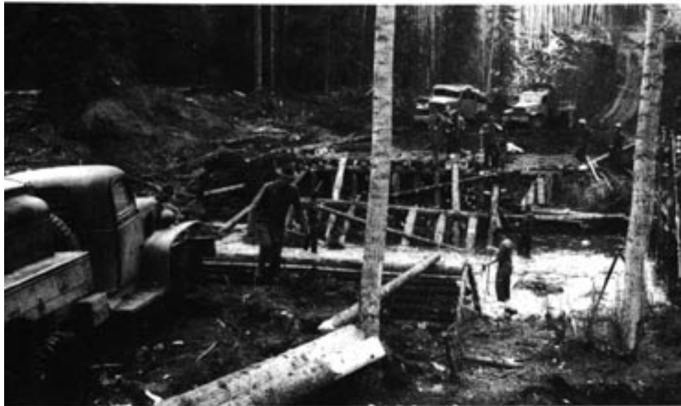
Cutting through the great North American wilderness in 1942, iron men and machines from the U.S. Army Corps of Engineers did their part in the war effort by constructing the Alaskan/Canadian Military Highway.
