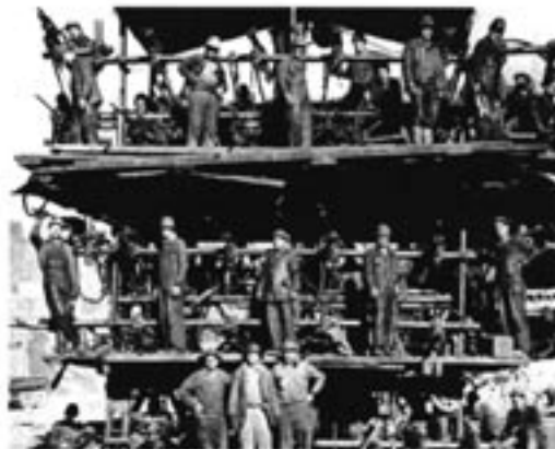
Boulder Canyon Project, Nevada, 1933.
