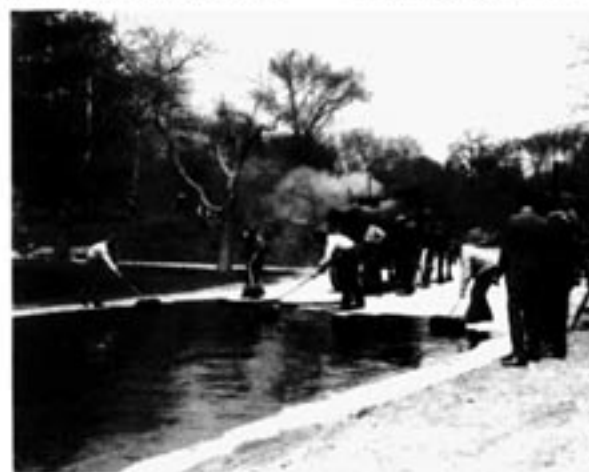
Spreading hot asphalt, ca. 1890s.
